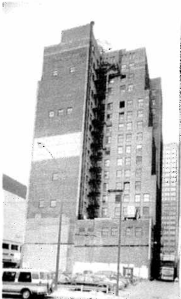
The building's west elevation was designed (left) so that another structure could be built behind it without blocking the light of most offices. The Grand Avenue facade (right) includes lower-level loading docks, sheltered by a classical-style balustrade.
